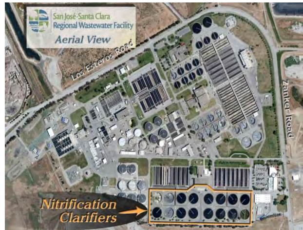
Figure 3 – Aerial View of Nitrification Clarifiers
