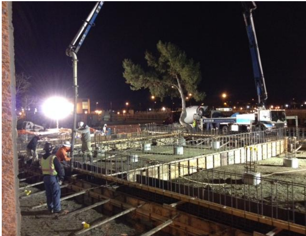
Figure 3: Grade Beams/Footings Concrete Pouring in Progress
