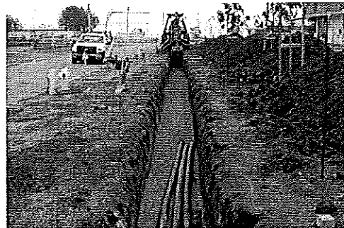
Fire Main Replacement - Phase 2
