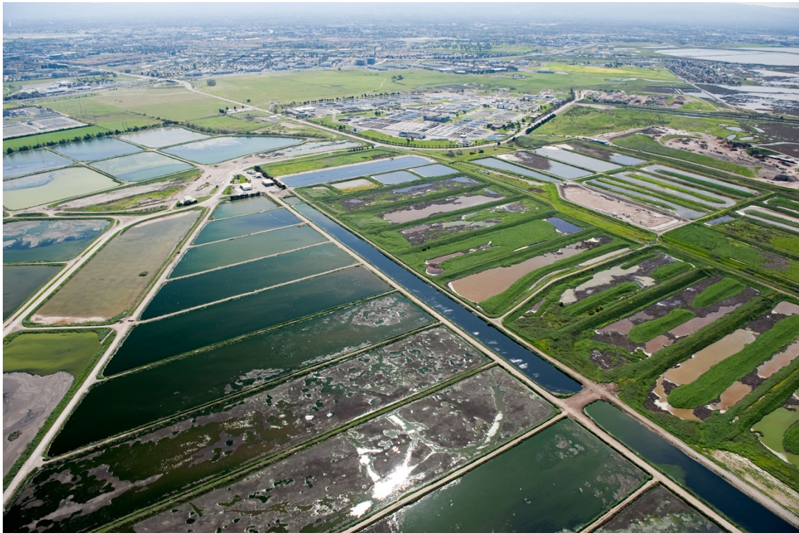
Figure 1 – By 2027, a new indoor, odor-controlled mechanical dewatering facility will be in place and the current outdoor biosolids sludge lagoons and drying beds de-commissioned (pictured here).
