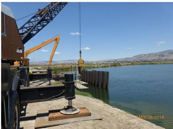
Piles and Pipes Installed, Headwall Installation Work
