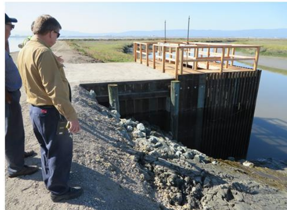
Completed Northern Gate Structure
