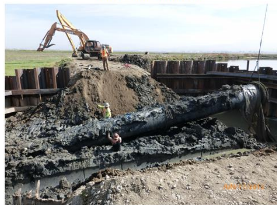
Removal of Pipes and Levee Material
