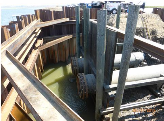
Piles and Pipes Installed, Headwall Installation Work
