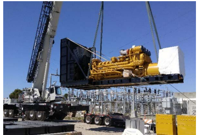
Figure 5 – Generator Engines Installation
