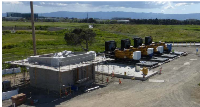
Figure 4 – Storage Building and Generators
