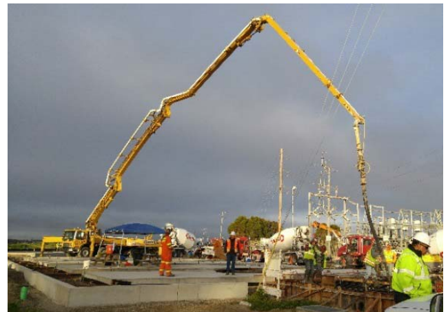
Figure 7 – Generator Concrete Pads Installation
