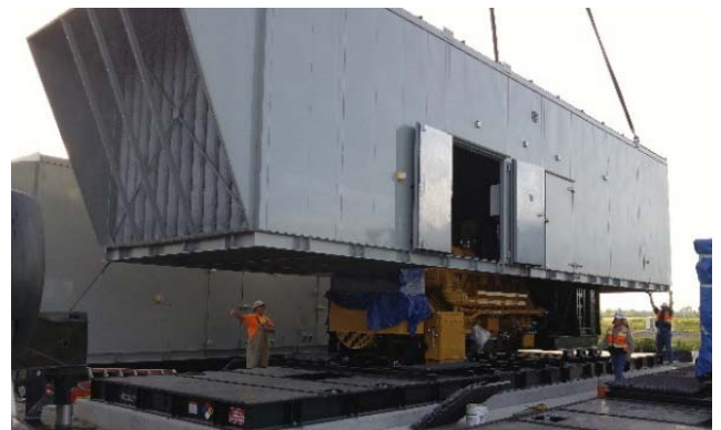
Figure 6 – Generator Enclosure Installation
