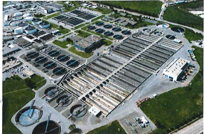
San José-Santa Clara Regional Wastewater Facility
