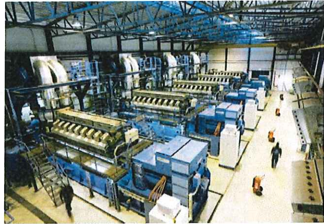
Internal combustion engines similar to the ones planned for the Cogeneration Facility
