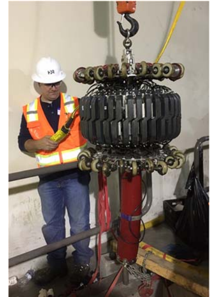
Figure 1: Technological devices such as the Pipeline Inspection and Condition Analysis' Seesnake allow visual and electronic inspection of flooded piping.
