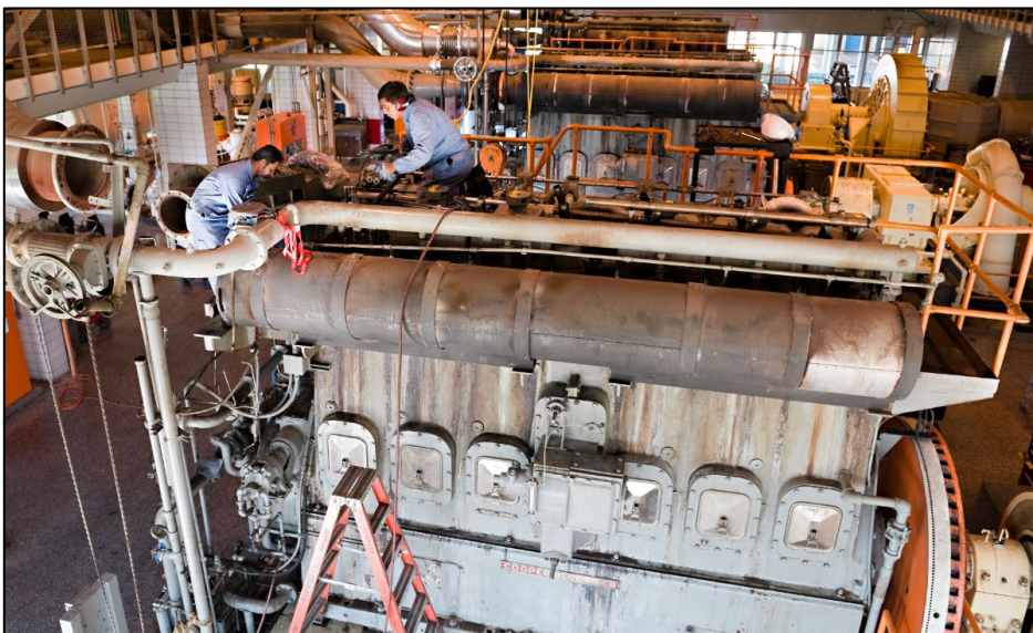
Cooper engine-driven blower SBB B-1 being serviced in 2014.
