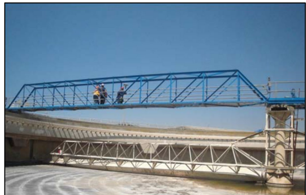
Worker on a clarifier “Tow-Bro” arm.
