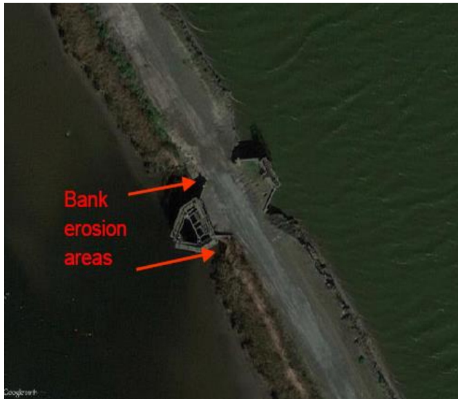
Figure 24. Bank erosion areas at the southern hydraulic structure
