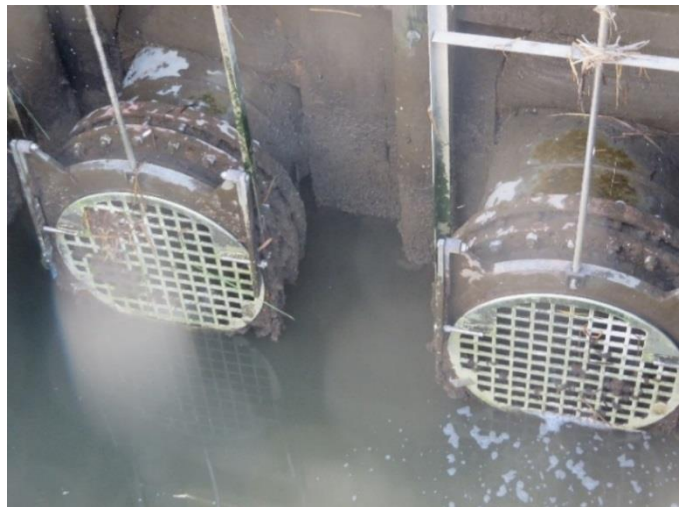
Figure 25. Steel flap gates were replaced with slotted fish screens to allow for inflow while preventing fish passage
