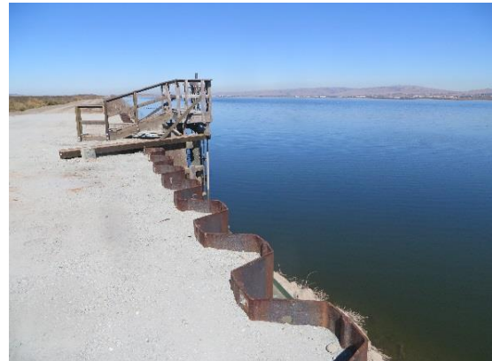
Figure 12. Pond A18 water color observations. Greenish-brown waters after flow regime reversal, 16 October 2018
