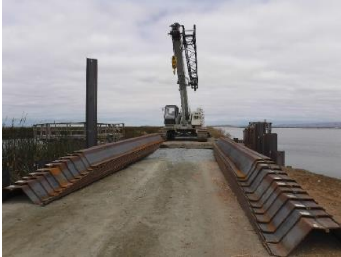
Figure 27. South Gate Levee Repair Project
