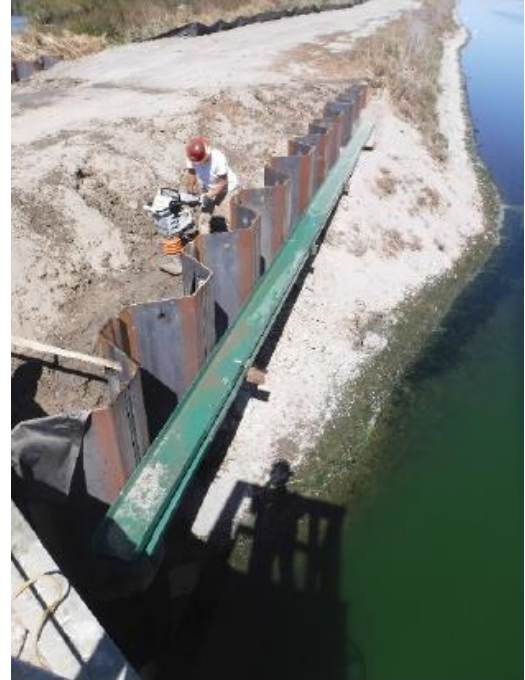
Figure 28. Walers affixed to sheet piles
