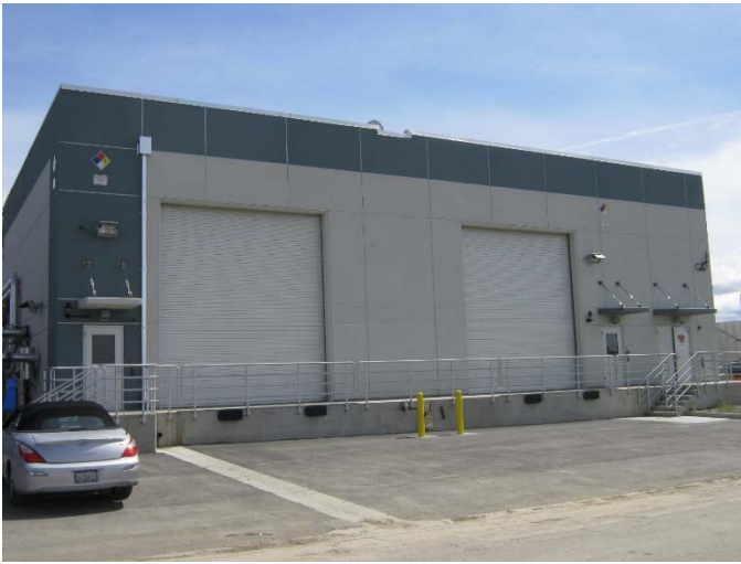
Figure 4: New Digester Gas Compressor Building
