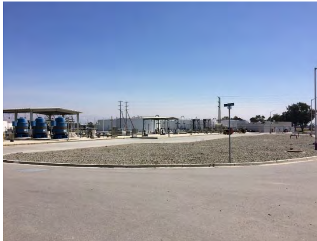
Proposed Site for New Headworks
