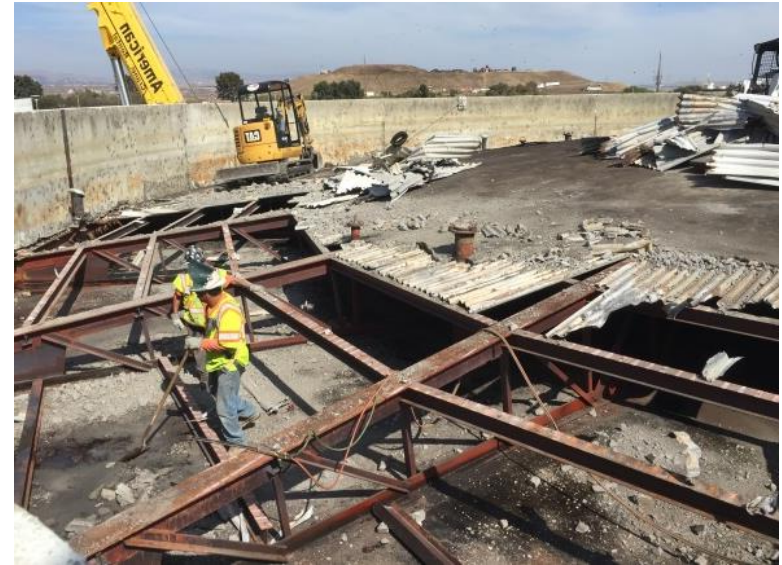
Digester & Thickener Facilities Upgrade
