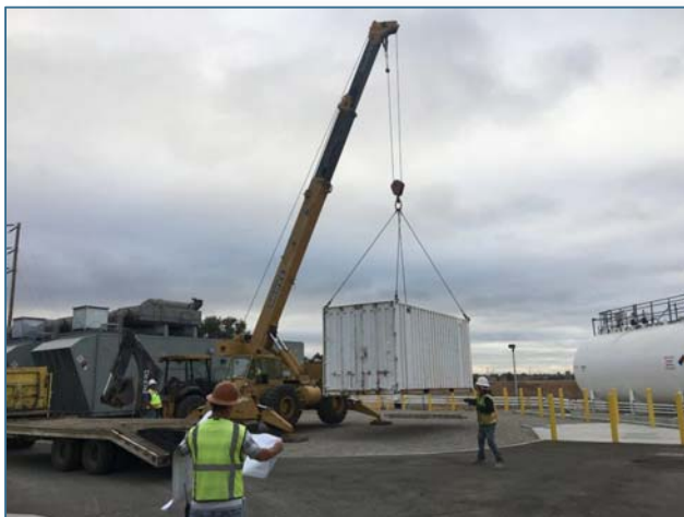
Figure 1: Inspectors on the job site
