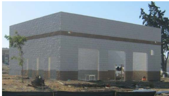
Figure 3: Partially Constructed Building
