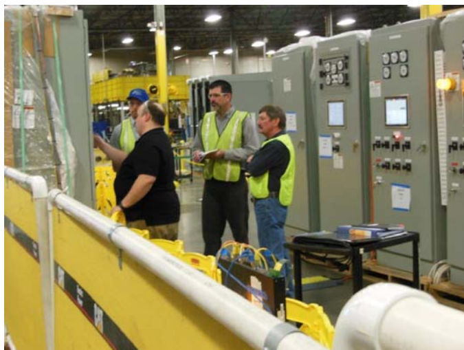
Figure 2: Emergency Diesel Generator FAT for the Switchgear and Control Panels
