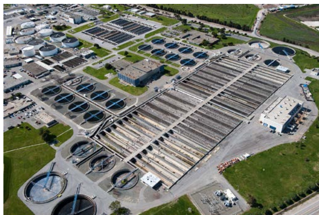
San José-Santa Clara Regional Wastewater Facility
