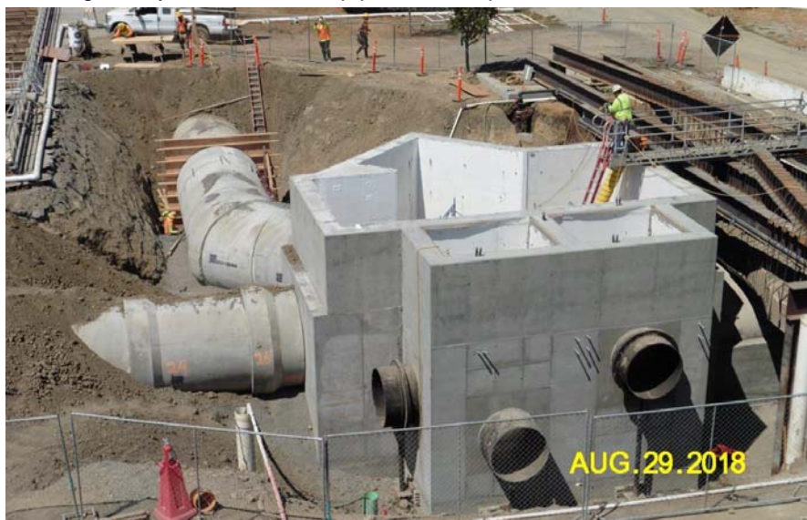
Figure 2: New wye structure
