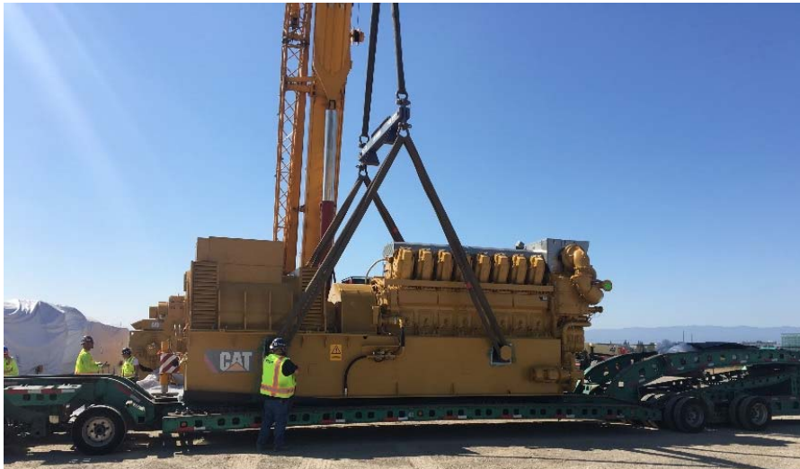
Figure 1: Unloading Caterpillar CG260-16 engines at the RWF
