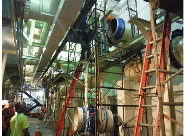
Figure 2: Existing valves in filter gallery to be replaced
