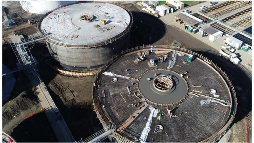
Figure 1: Digester 6 Concrete Roof Under Construction, Digester 5 Roof Completed
