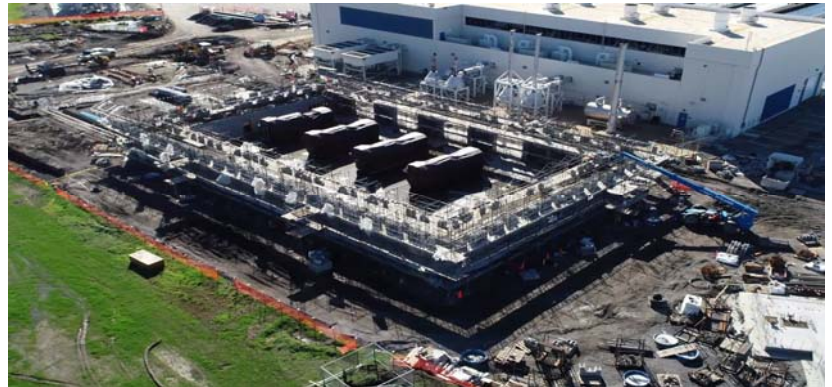
Figure 1: CMU wall construction at the new cogeneration building.
