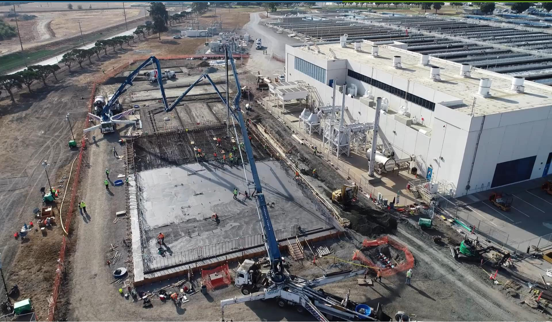
Cogeneration Facility – Building Pad A & B Concrete Pour
