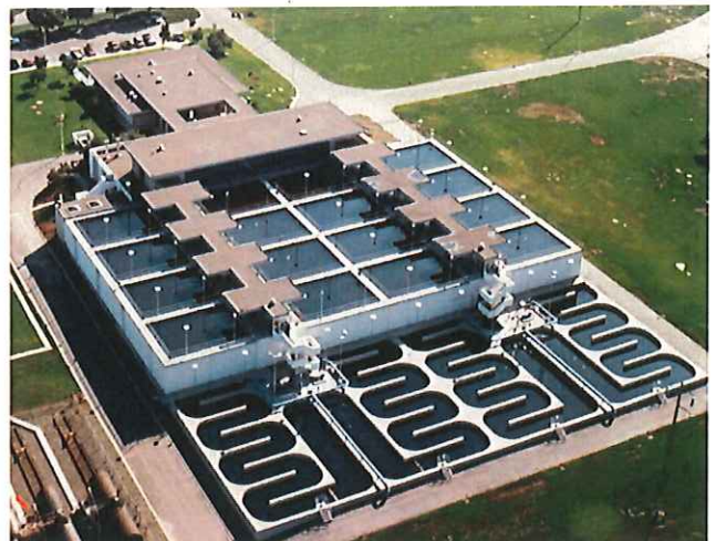
Aerial of Filter Building
