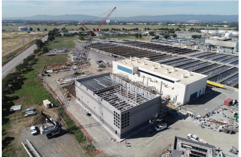
Figure 1: Cogeneration Main Generator Building roof truss installation
