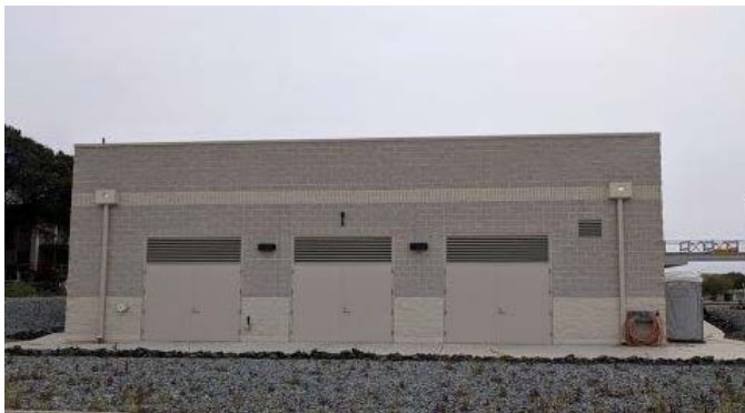
Figure 8: New Plant Air Compressor Building
