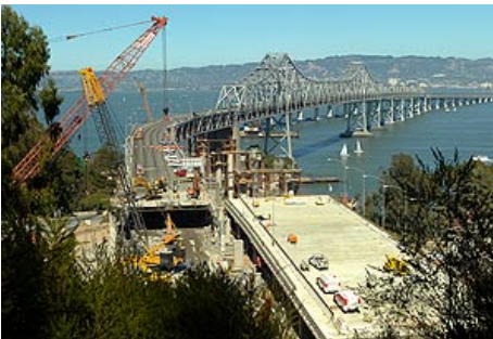
Bay Bridge deck replacement
