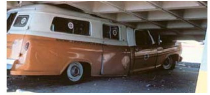
Hospital parking structure collapse crushes ambulance
