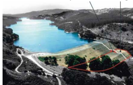
San Pablo Dam and Reservoir Upgrade
