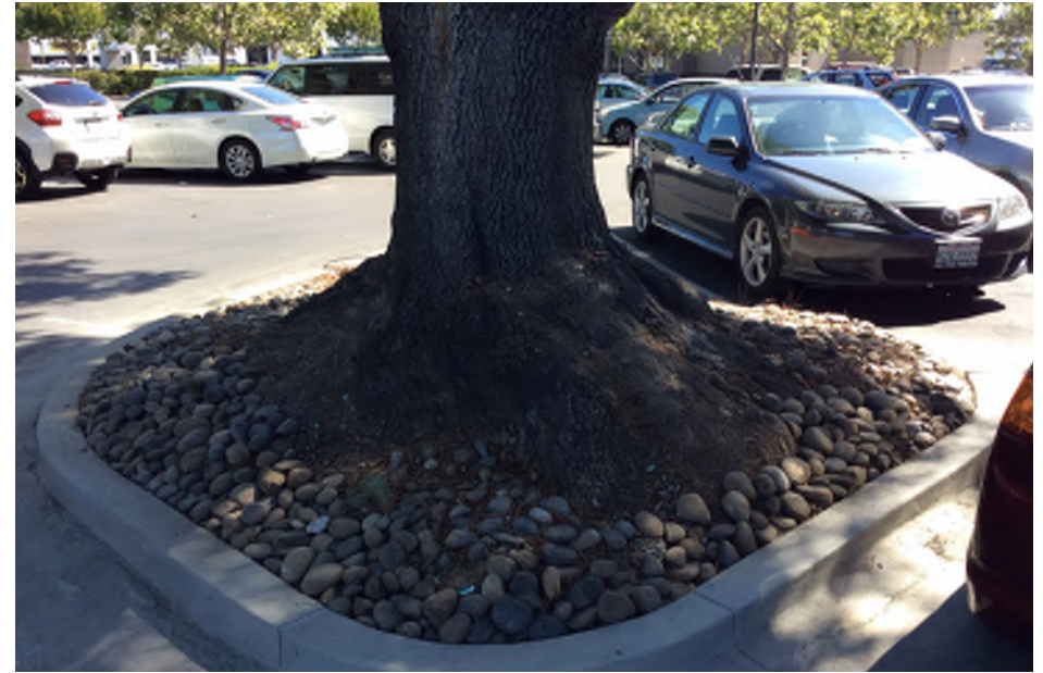
Recently repoured curb may have impacted root zone.
