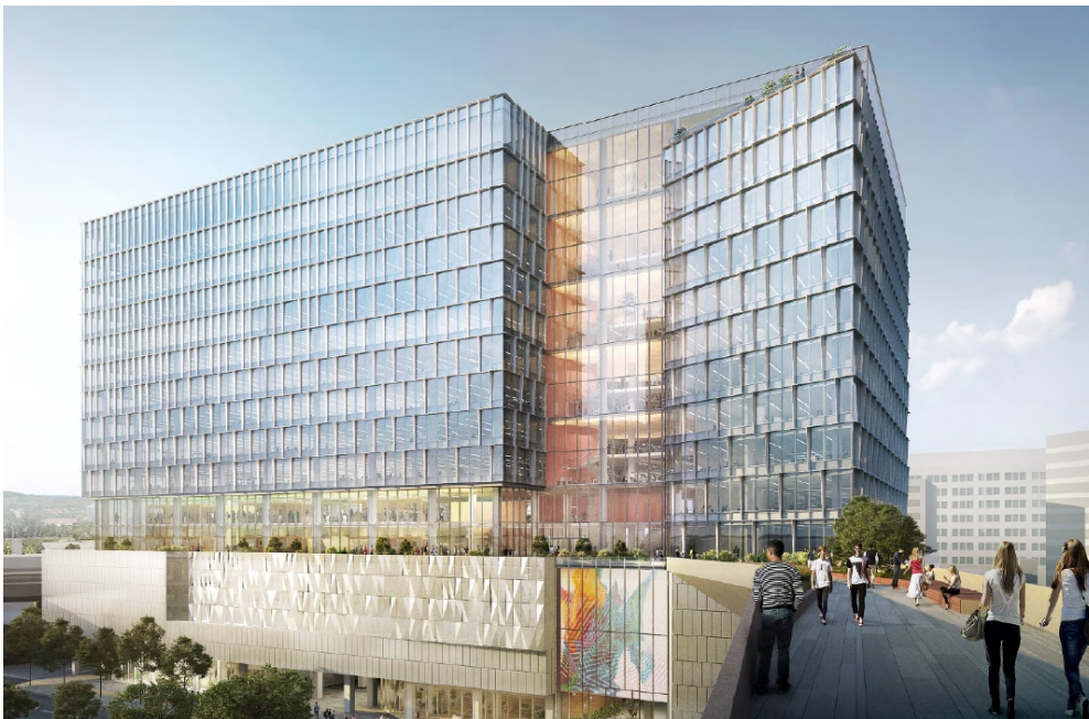
Figure 4. Bird collisions with the curtain wall in the alcove may be greater due to the clear glass panels without spandrels and the vegetation shown on the inside of the building. In addition, glass railings along the edge of the 17 th floor green roof will pose collision hazards to some extent.
