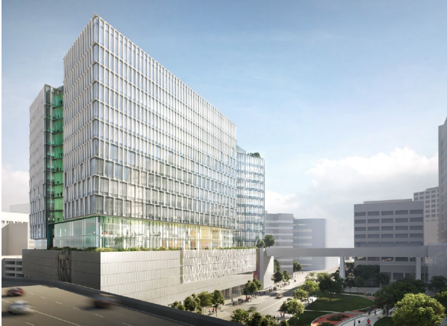
Figure 3. The façades of the Adobe North Tower are composed primarily of glass, but vertical and horizontal louvers and spandrel panels break up the façades on most of the proposed building to some extent. Opaque panels are present over the garage levels.
