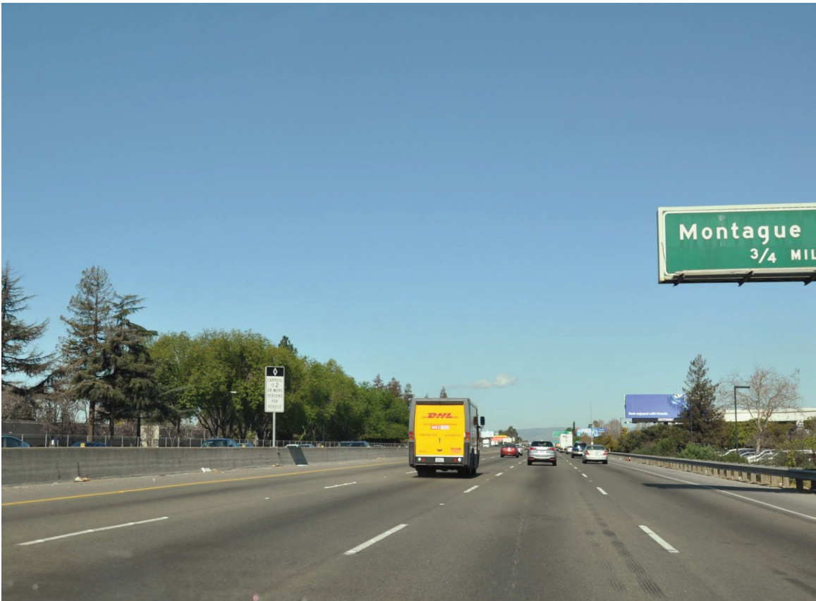
Photo 2: View of I-880 looking north.
