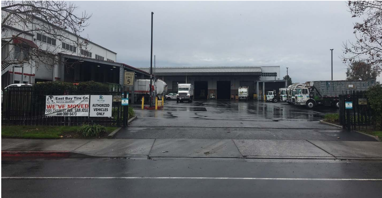
Figure 6. Photograph of Site (North Entrance)
