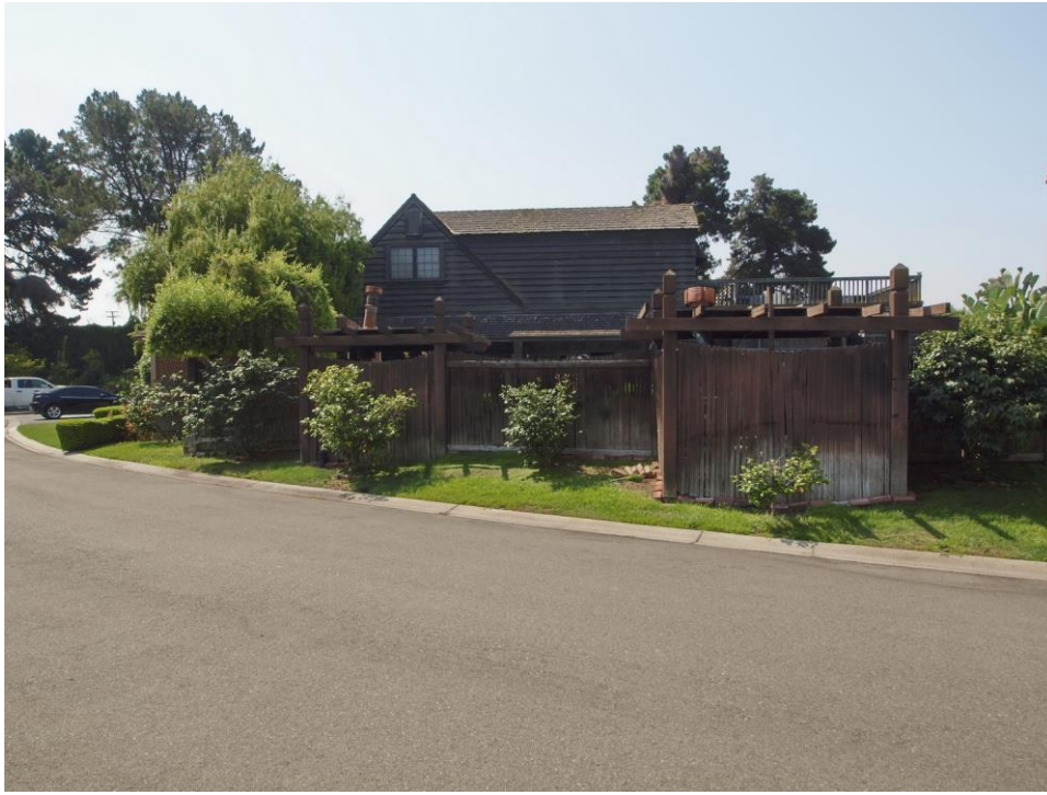
Community Center building, facing south.
