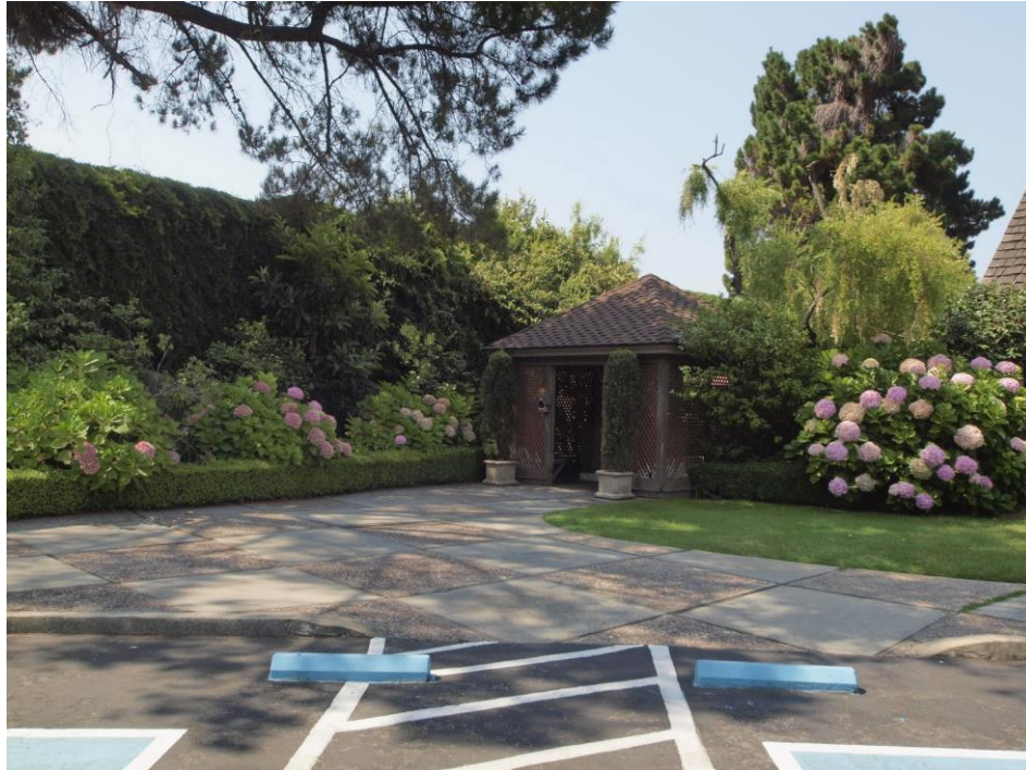
Entry to Community Center from east through pump structure from Winchester estate.
