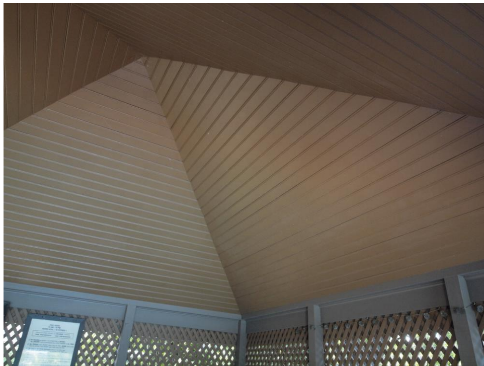
Inside ceiling of spa structure.
