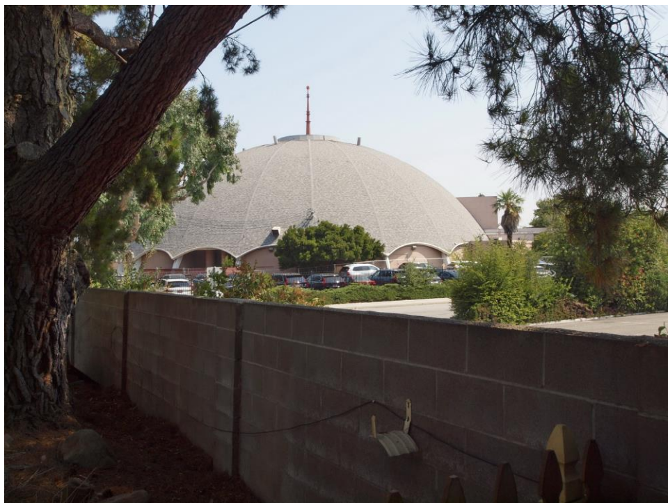
Century 21 Theater beyond northeast property fence, viewed facing northeast.
