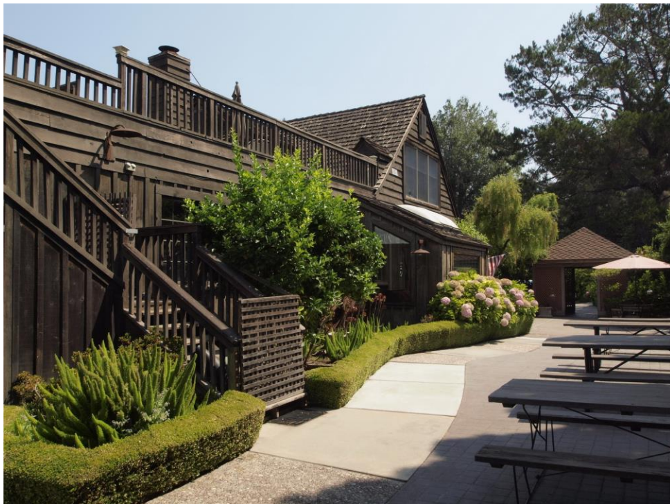
Community Center Building at south elevation, viewed facing east.
