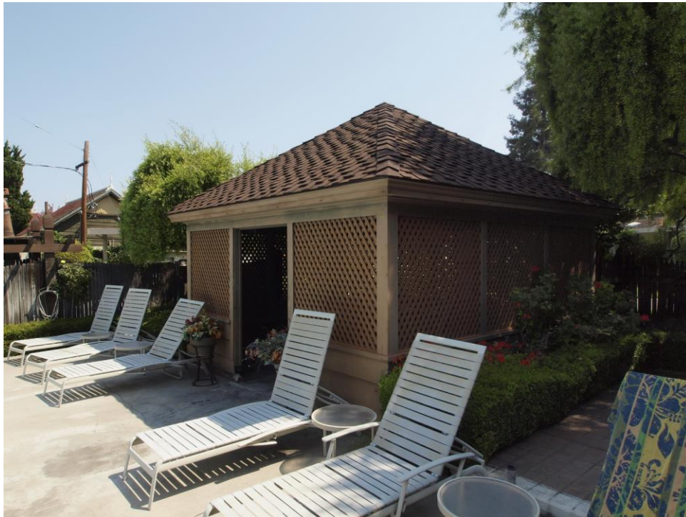
Spa structure at pool consisting of relocated pump structure from Winchester Estate.
