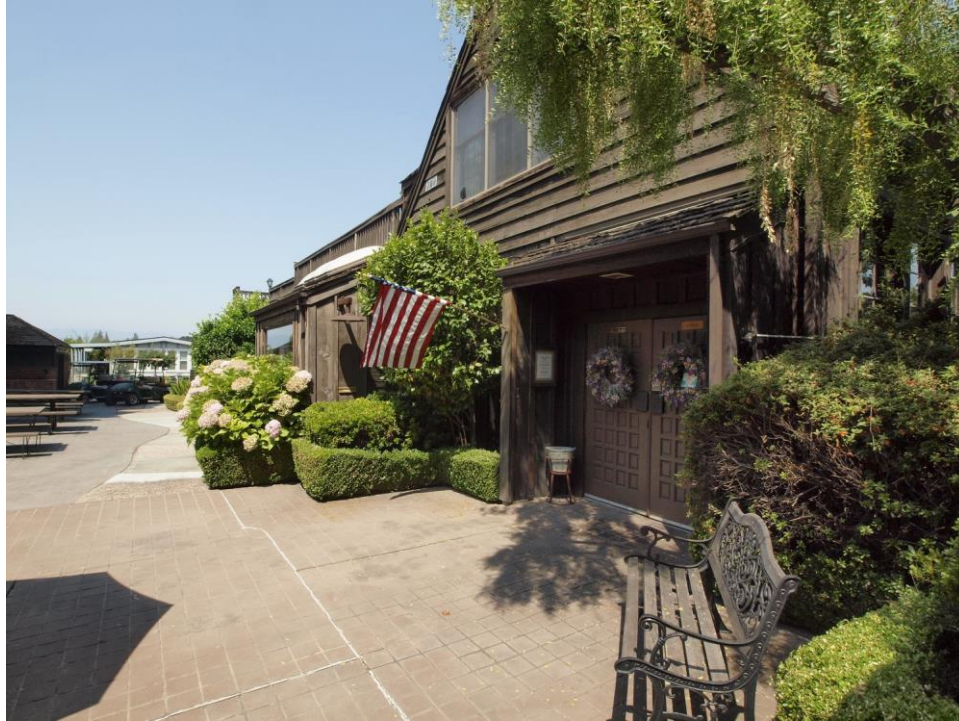
Community Center building at south elevation, viewed facing west.
