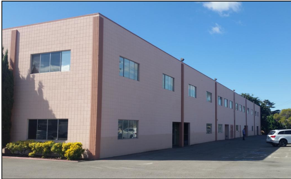
Figure 3. Northeast corner and north (rear) elevation.
