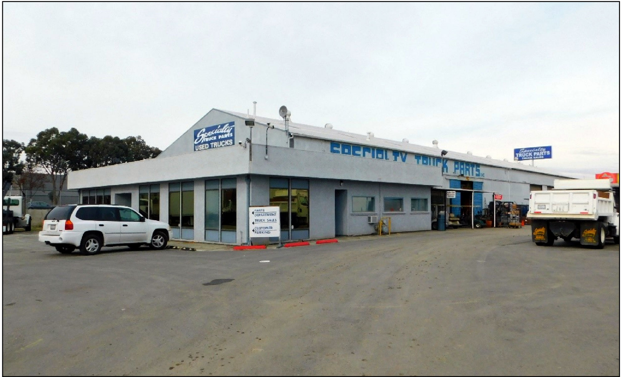
Photo 5: Looking northwest from the Industrial Avenue entrance
