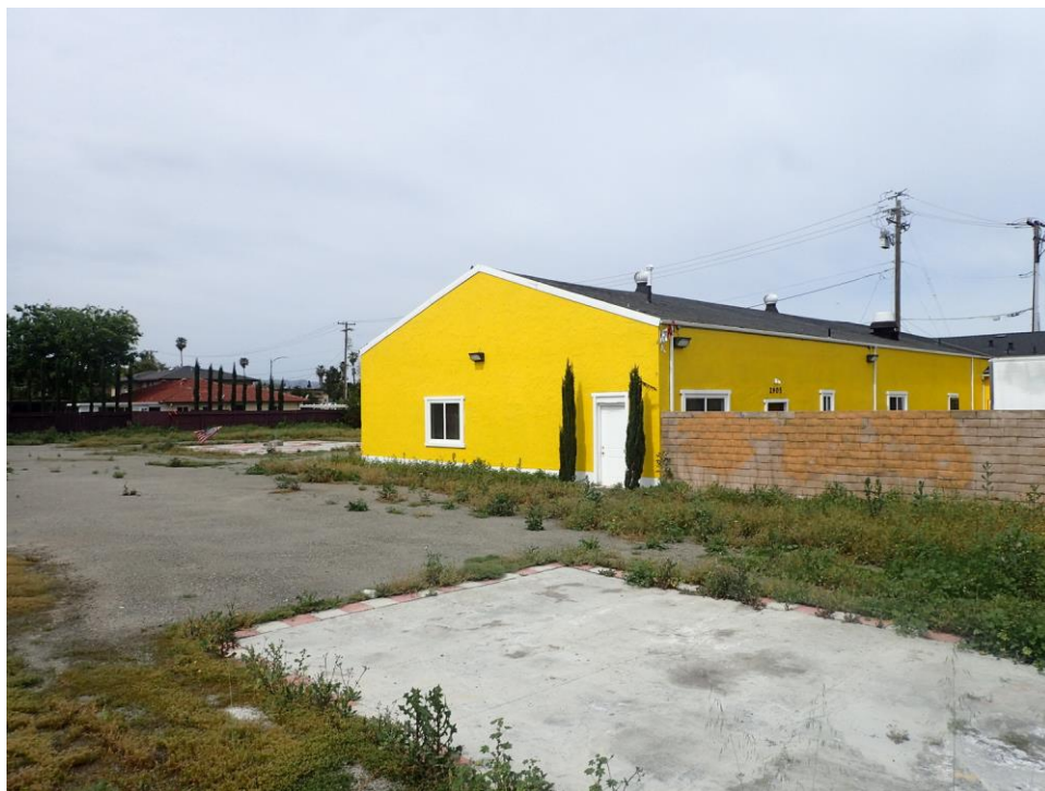
South side of 1960s building, viewed facing northwest.
