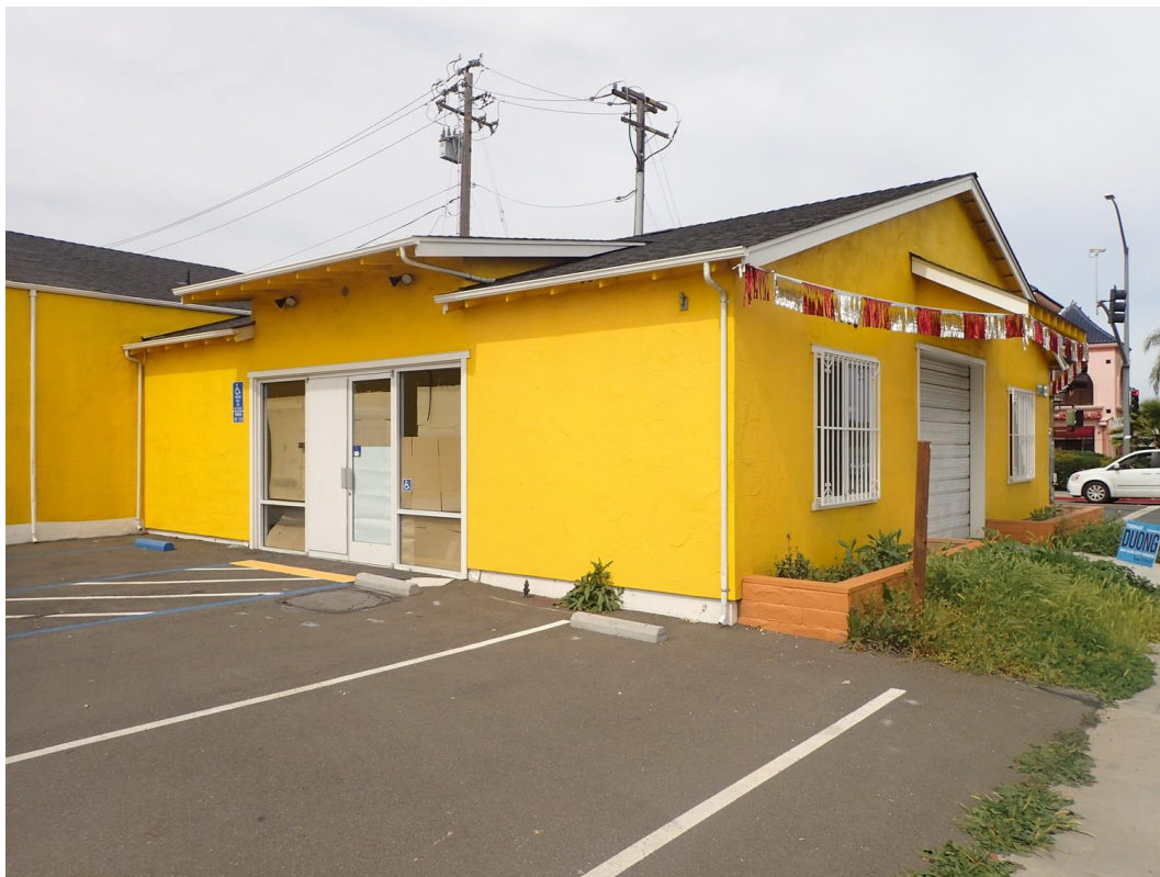
Main entry at parking area of front building, viewed facing northwest.
