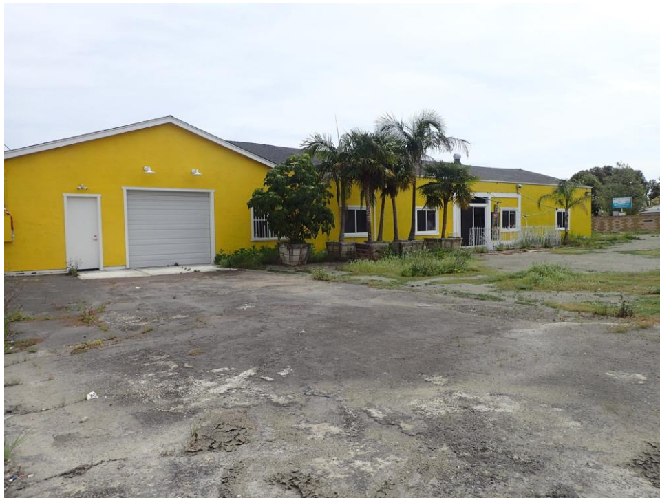
Rear of site from Lewis Road, viewed facing southeast.
