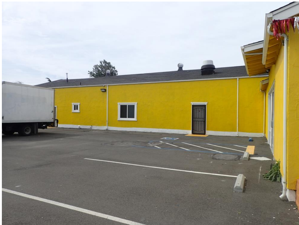
Front parking area with 1960s building to rear, viewed facing southwest.
