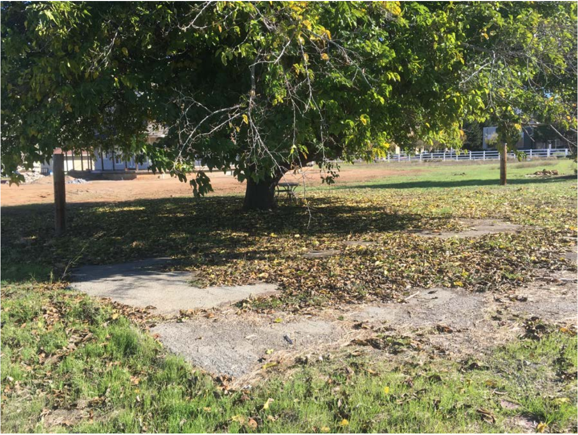
Photograph 3 - Concrete poured on Property
