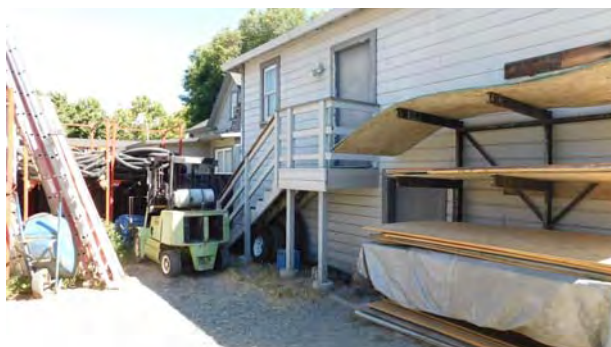
Rear portion of the main house
