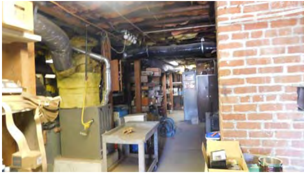
Ground level garage within the 1452 residential structure
