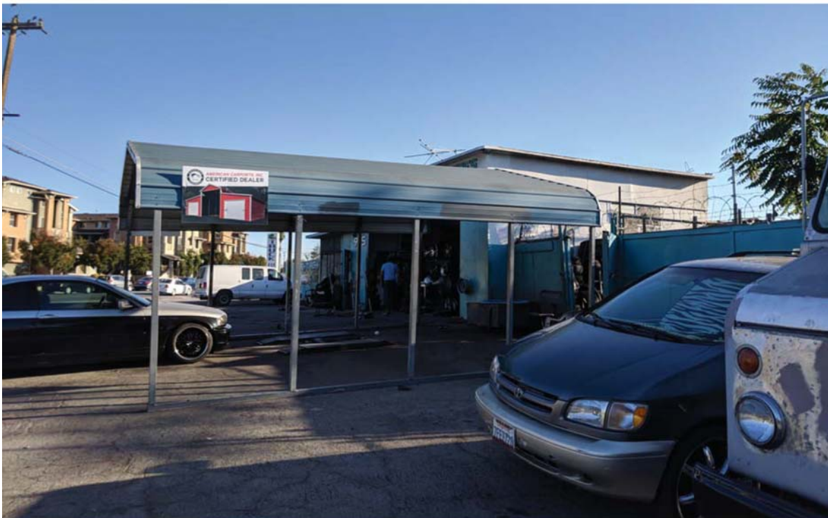
Photo 2: View of tire repair shop looking southeast from driveway at Horning Street
