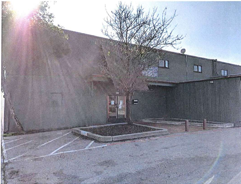
Photo SE-1: View of commercial buildings south of project site from site's southeast corner.
