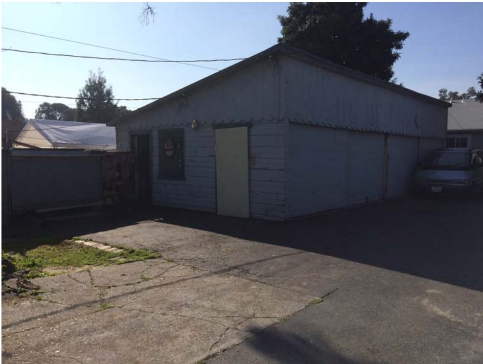
Photo 2: Garage converted to two storage units.
