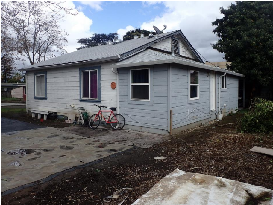
Rear dwelling from backside, viewed facing northeast.
