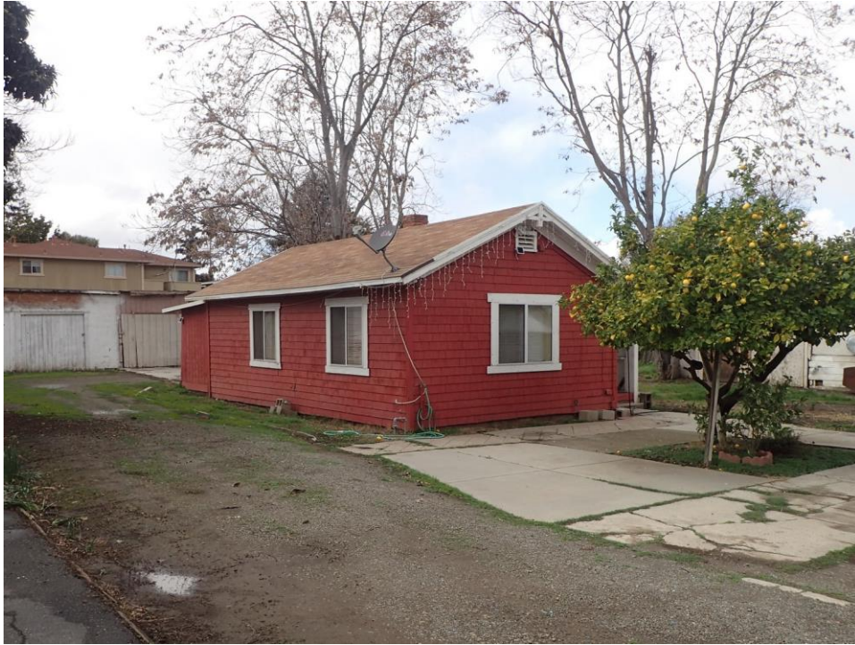
Small secondary dwelling unit, viewed facing west.
