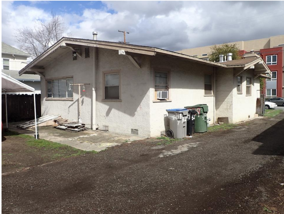
View of rear of house facing north.
