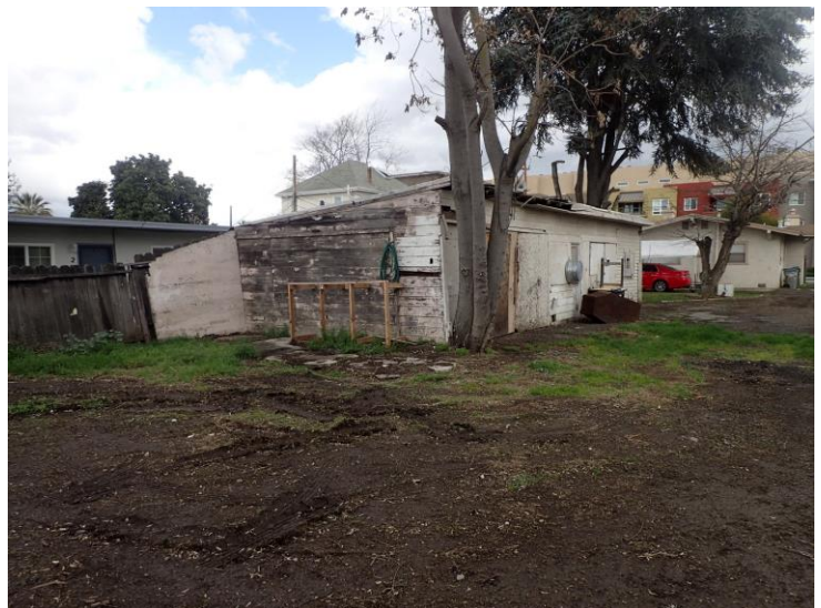
Garage structure viewed facing northeast
