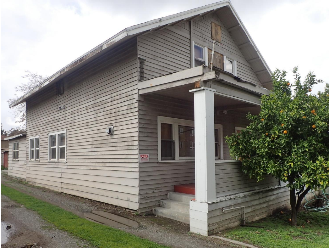
View facing west showing front porch and driveway.
