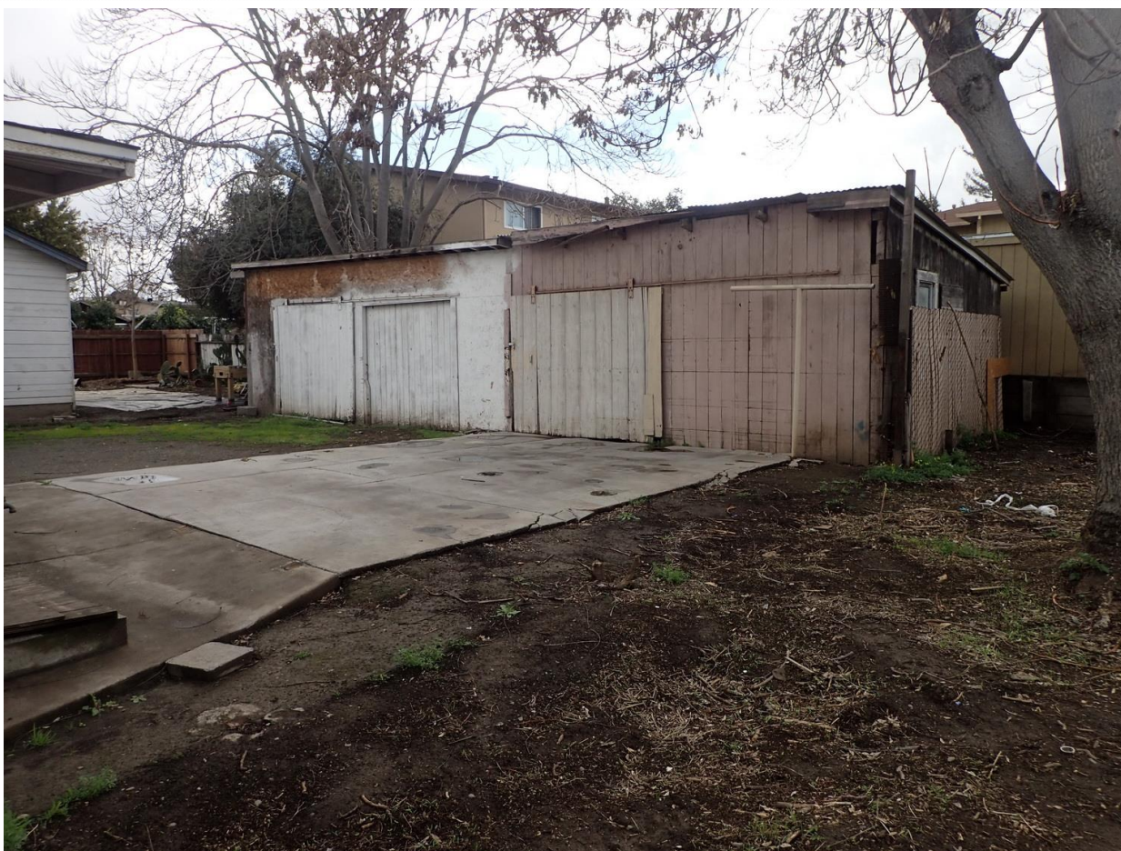
Rear garage on right, viewed facing southwest.
