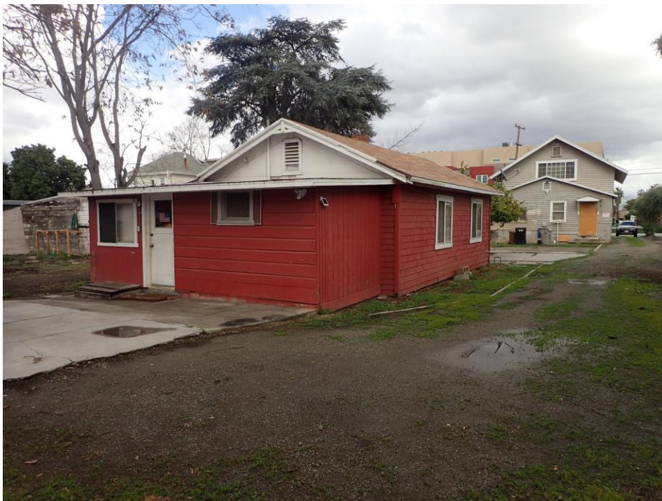
Secondary dwelling unit from rear, viewed facing northeast with main house in distance.
