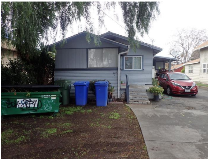
Front house from Page St. viewed facing west.
