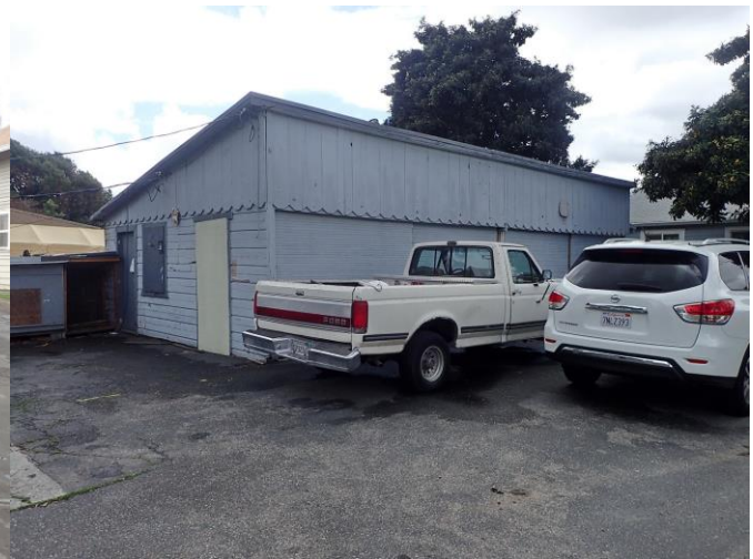
Garage at mid-site, viewed facing south.
