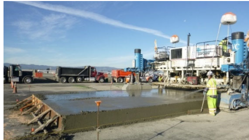
Terminal B Ramp Rehabilitation
