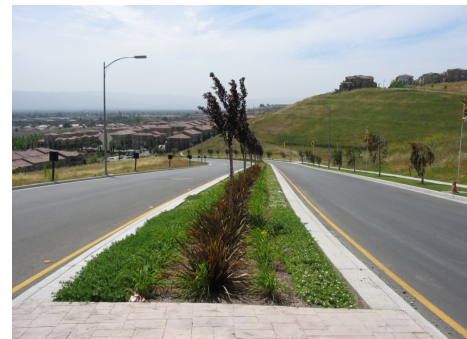
Median Island at Communication Hill
