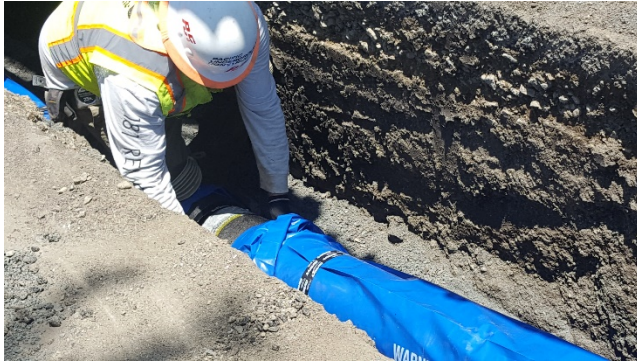
Installation of New Pipe at Gumdrop Drive
