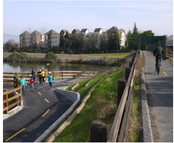
Coleman Road Under-crossing
