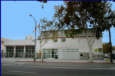
Major Repairs at Fire Stations 3, 4, 9, 14 and 30
