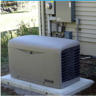
A hard-wired generator must be installed on a concrete pad.
