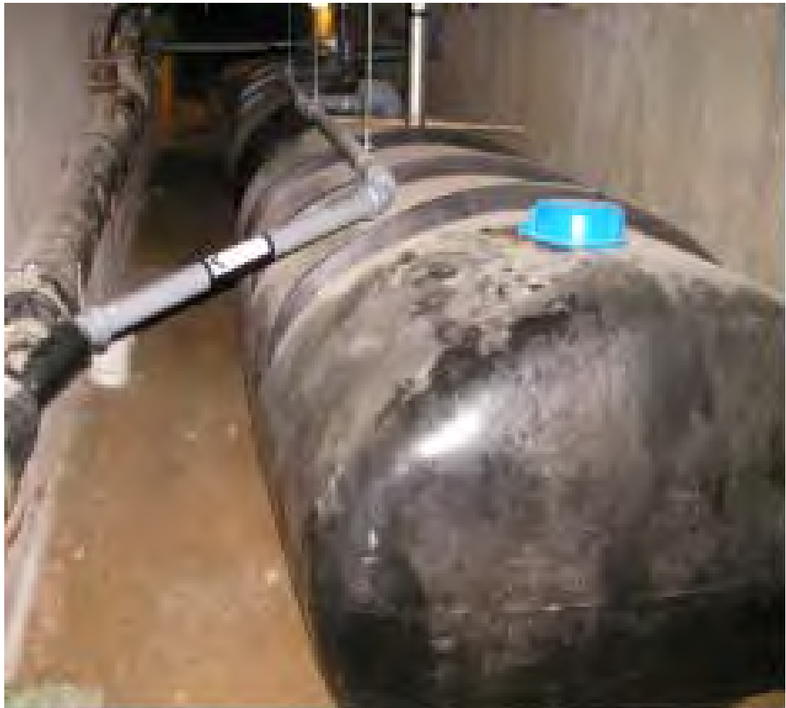
Figure 7 Typical Long-Term Urine Storage Tank. Source: Follner, 2008
