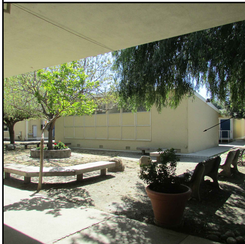
BUILDING 18 (TO BE DEMOLISHED) LOOKING SOUTH
