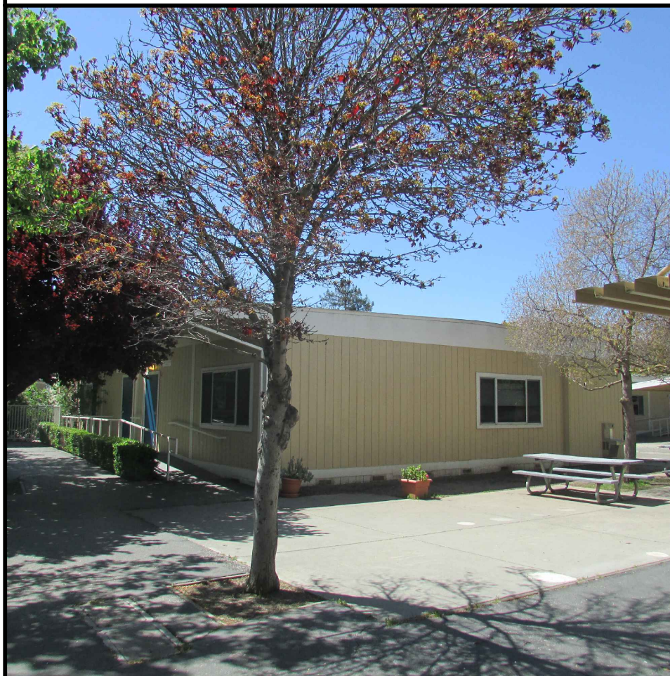
BUILDING 20-21 LOOKING SOUTH
