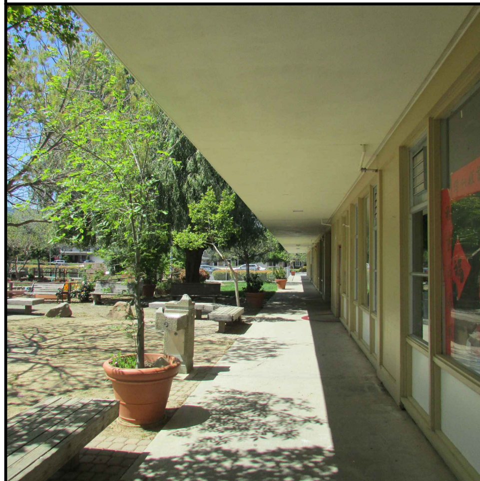
CLASSROOM BUILDINGS LOOKING WEST
