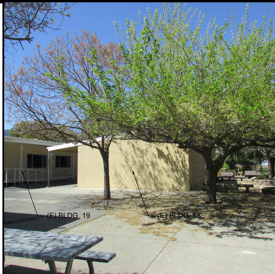
BLDG 19 AND 18 LOOKING WEST
