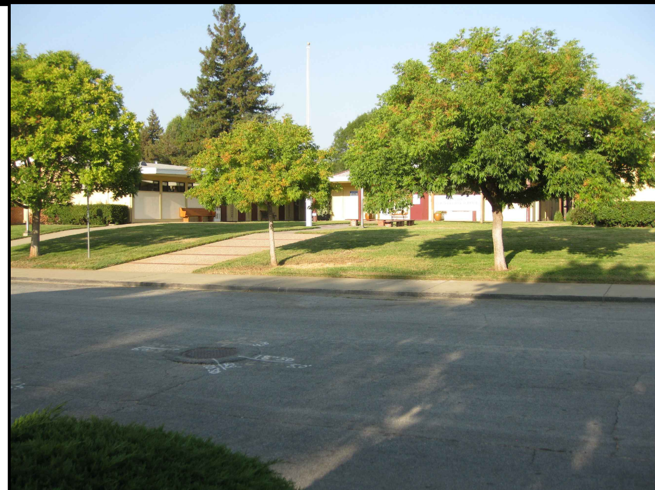
ADMINISTRATION BLDG. OFF TRINIDAD DR.
