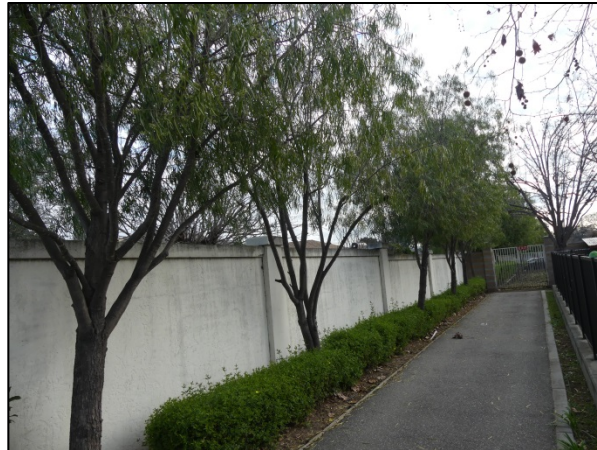
Photo 2. Looking along the north property line.
