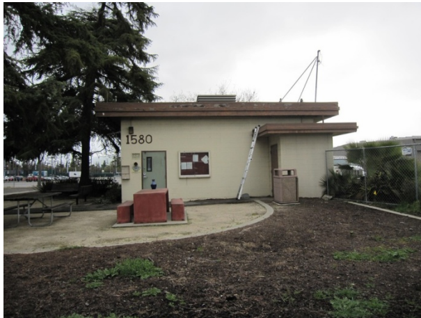
Photograph 1. View of the on-site building looking east.
