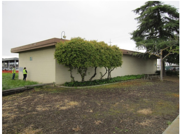
Photograph 2. View of the on-site building looking southwest.
