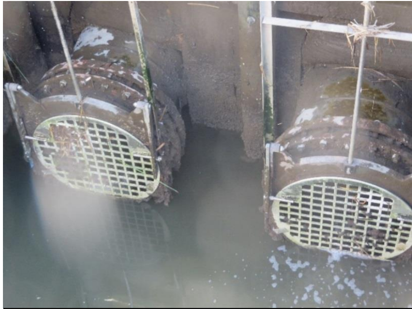
Steel flap gates were replaced with slotted fish screens to allow for inflow while preventing fish passage.
