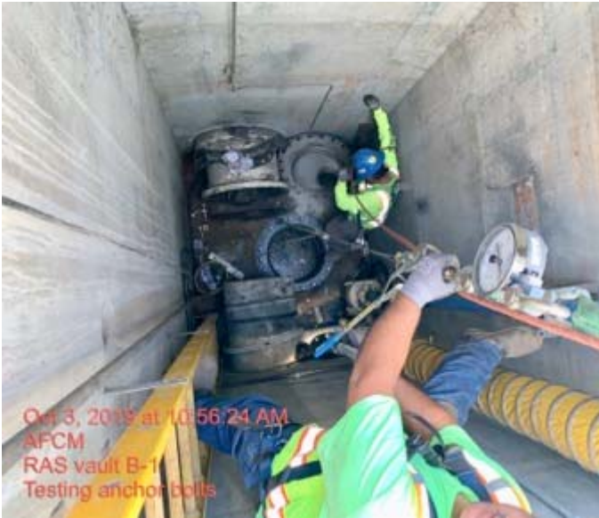
Figure 5: Ongoing Secondary Return Activated Sludge Magnetic Flow Meter Work
